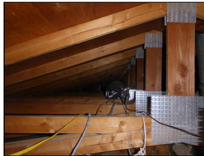
Attic - Engineered Truss System
