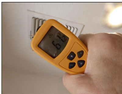
Unit 2 - Supply Air Temp
