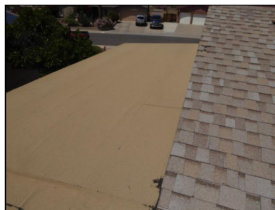
West Shed Roofing
