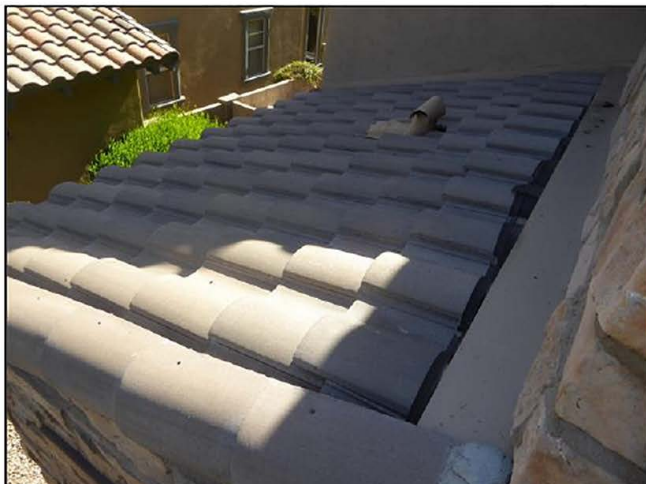
Roof - North facing (1st level)
