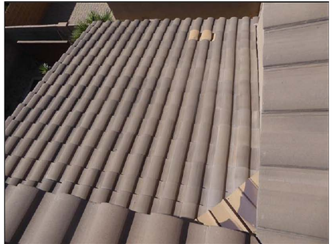
Roof - East facing (1st level)
