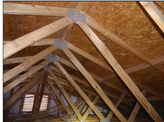
Attic - Engineered Truss System
