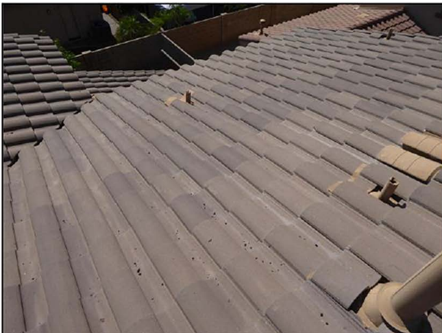
Roof - East facing (R)
