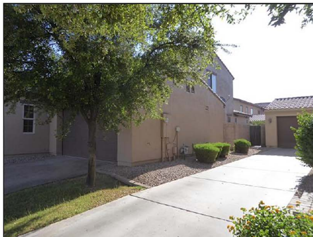
Exterior - South exposure
