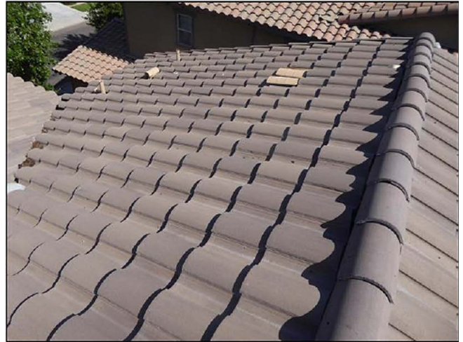
Roof - North facing (L)
