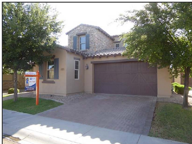
Exterior - West exposure
