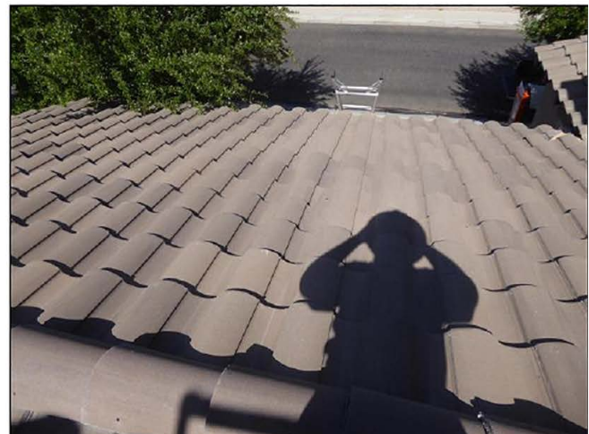
Roof - West facing (1st level)
