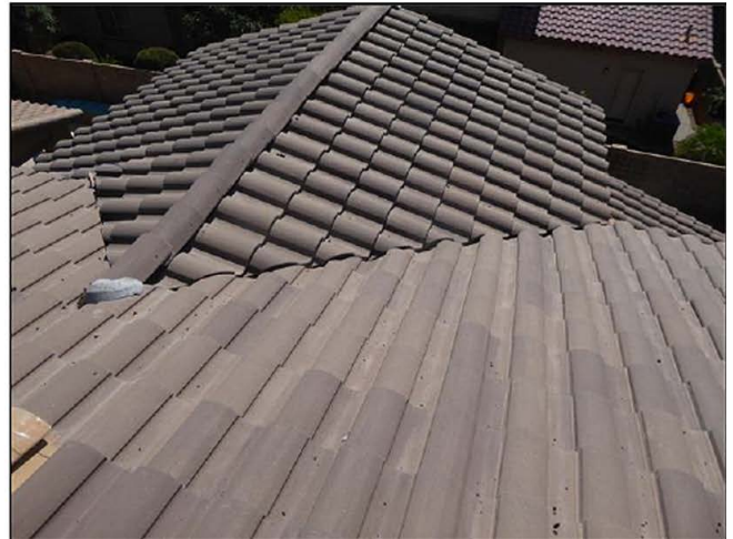
Roof - East facing (L)
