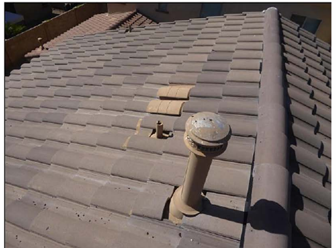
Roof - South facing (L)
