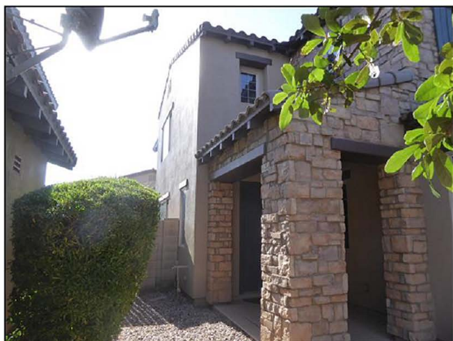
Exterior - North exposure
