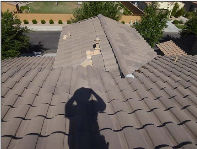
Roof - West facing (R)
