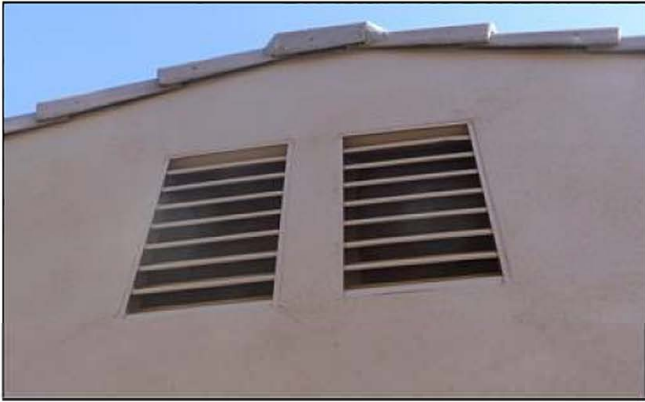
Attic - Gable Vents
