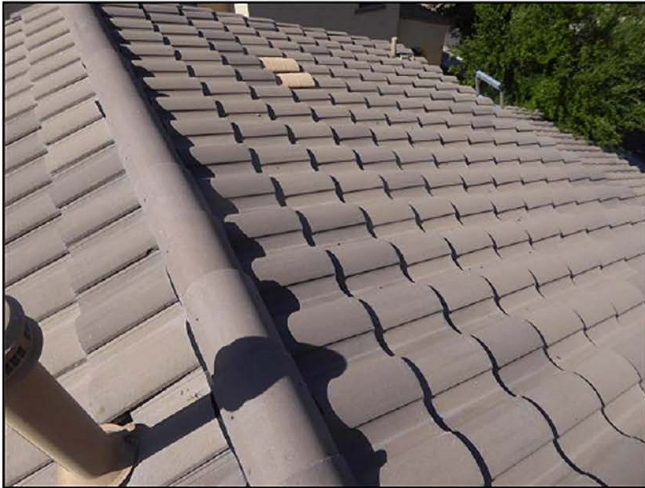
Roof - South facing (R)
