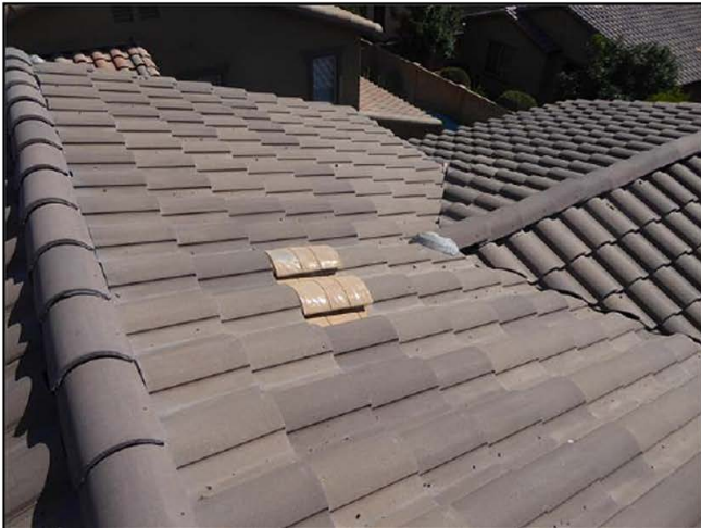
Roof - North facing (R)
