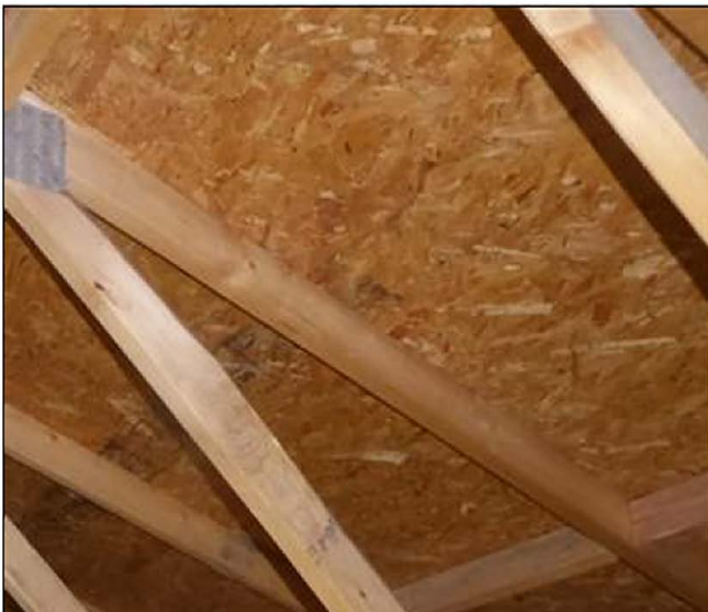
Attic - OSB Sheathing
