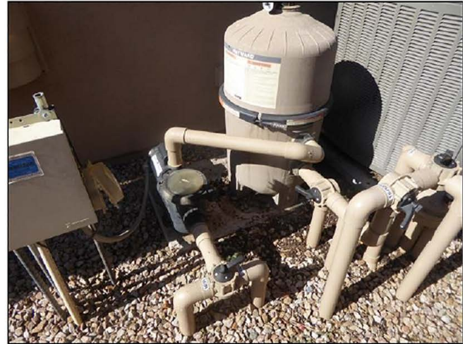
Pump/Filter System
