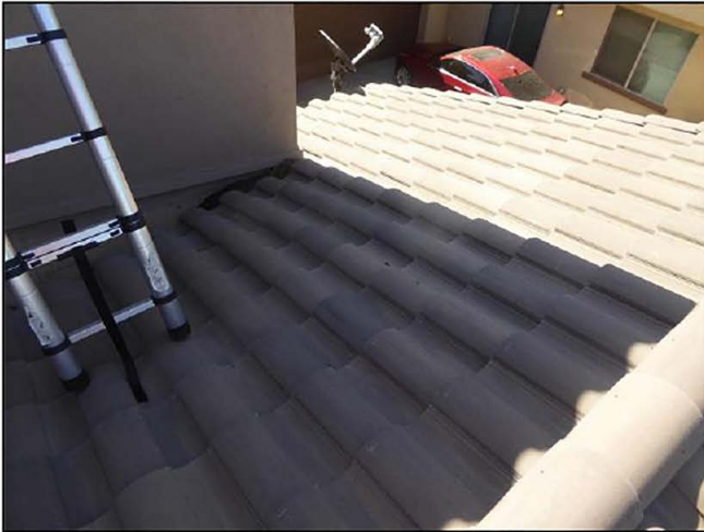
Roof - South facing (1st level)
